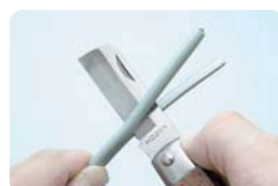
VVF wire's jacket stripping
